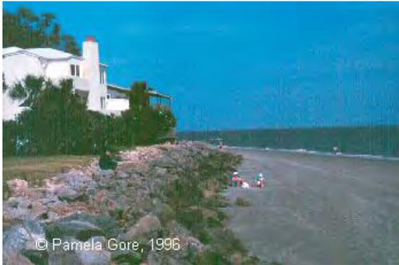
the base and over sweep erodes the back of the barrier. No new natural dune creation has occurred from the time the barrier rocks were installed. There have been numerous isolated permitted attempts to reestablish the primary dune through use of manmade biodegradable sand bags and sand tubes incorporating native vegetation. Sea Island has been more successful in maintaining the
